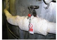
some other means used to indicate that they are not to be opened and notices placed on the relevant controls. The officer on watch should be informed.
