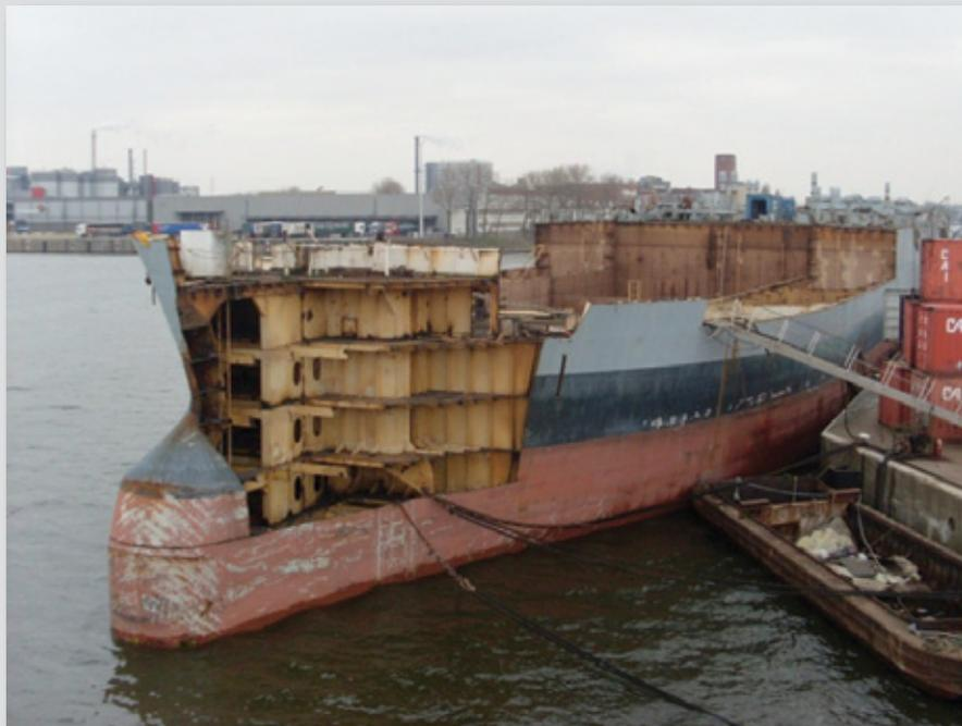
3 photos showing superstructure completely removed, the Engine room opened up and the first "layer" of the ballast/diesel tanks almost all removed
