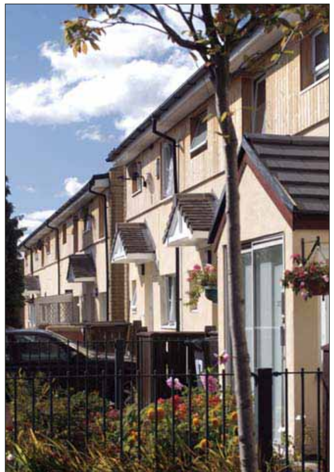
Newly refurbished home at Grove Village, Manchester, made possible by the Housing Private Finance Initiative
