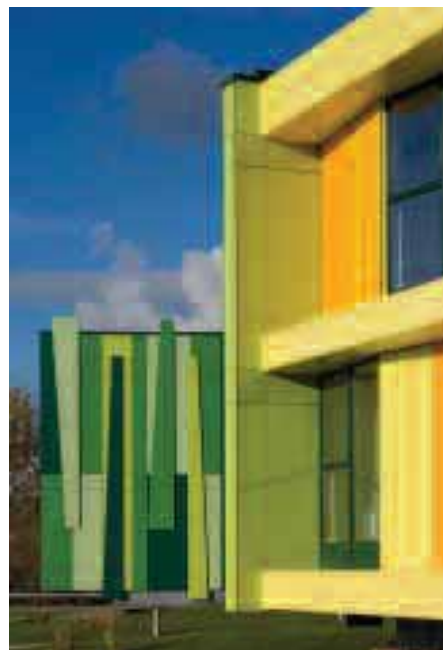
emda -funded Blueprint is accelerating regeneration in urban areas
