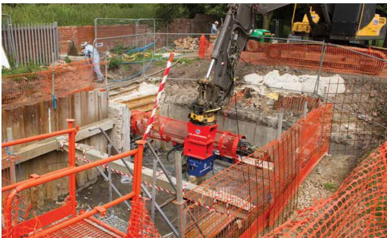
**Horizontal drilling operation to enable a former colliery subway in South Yorkshire to be grouted.**
