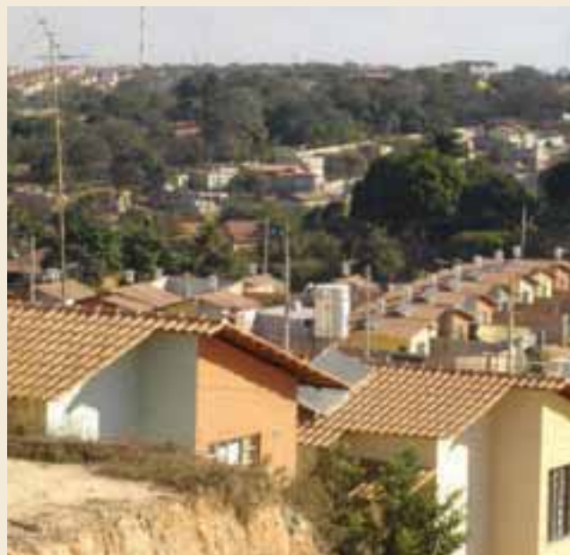
Solar panels in low income houses in Betim
