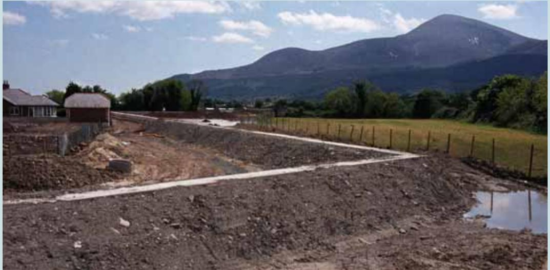
The scheme comprises 3,200 tonnes of steel sheet piles along with 3,000 cubic metres of reinforced concrete floodwall providing 3,300 metres of flood embankment along the riverbanks. In addition footbridges at 3 locations will be reconstructed and fisheries enhancement measures will be carried out.
