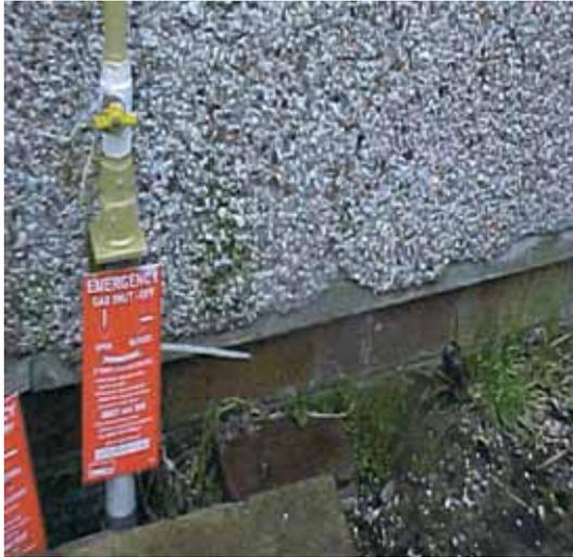
Figure 15 – Typical Emergency Control Valve (ECV) on outside of property
