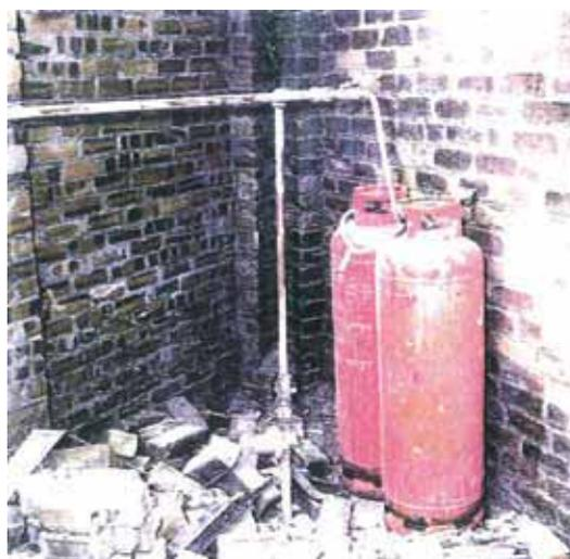
Figure 22 – The two manifolded 47kg propane cylinders
