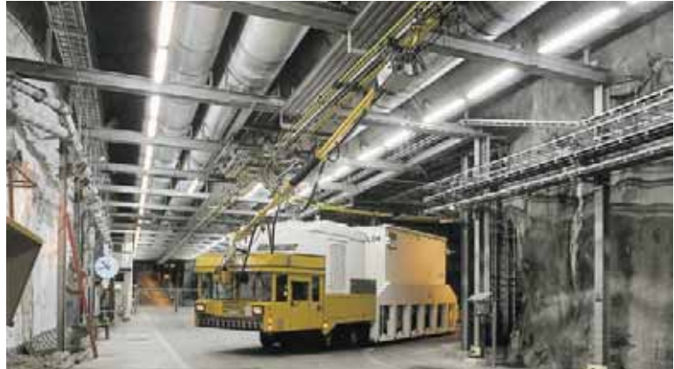
Underground transport facilities at a disposal facility in Sweden (courtesy SKB)
