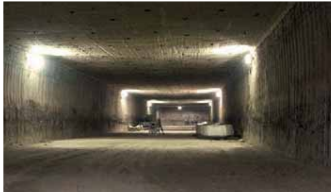
Underground facilities at the Waste Isolation Pilot Plant (WIPP) in New Mexico USA (courtesy WIPP information centre)
