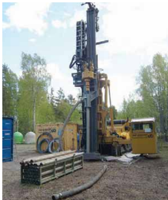
Borehole drilling during surface investigations in Sweden (courtesy SKB)
