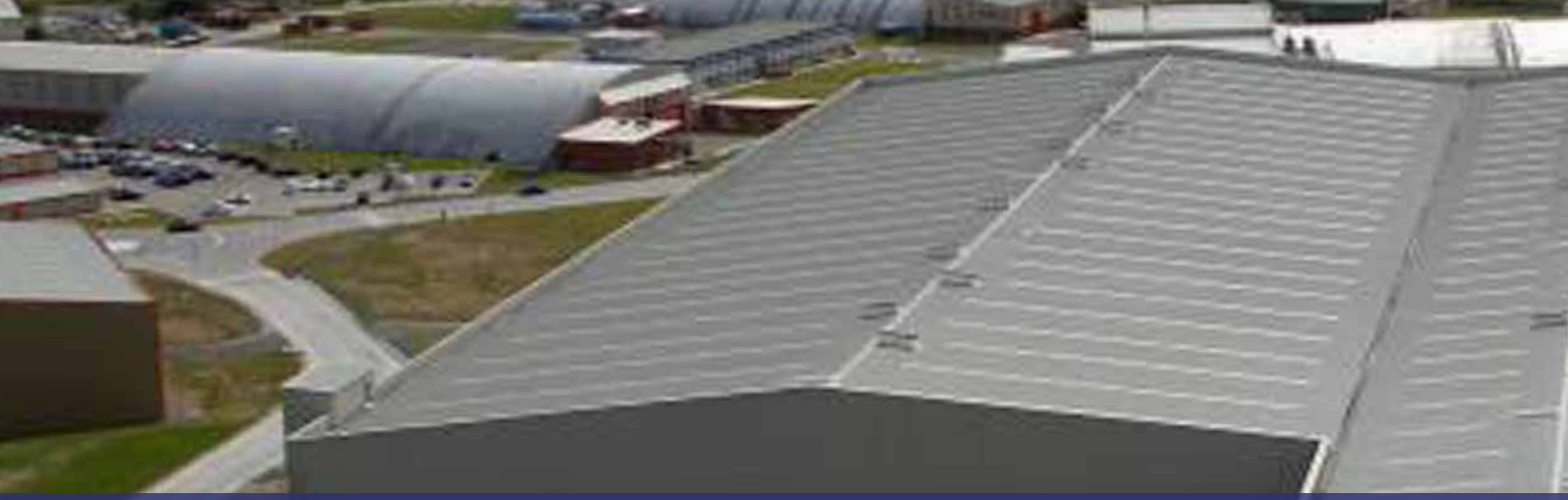
Airbus state of the art composite wing manufacturing facility in Broughton, Wales
