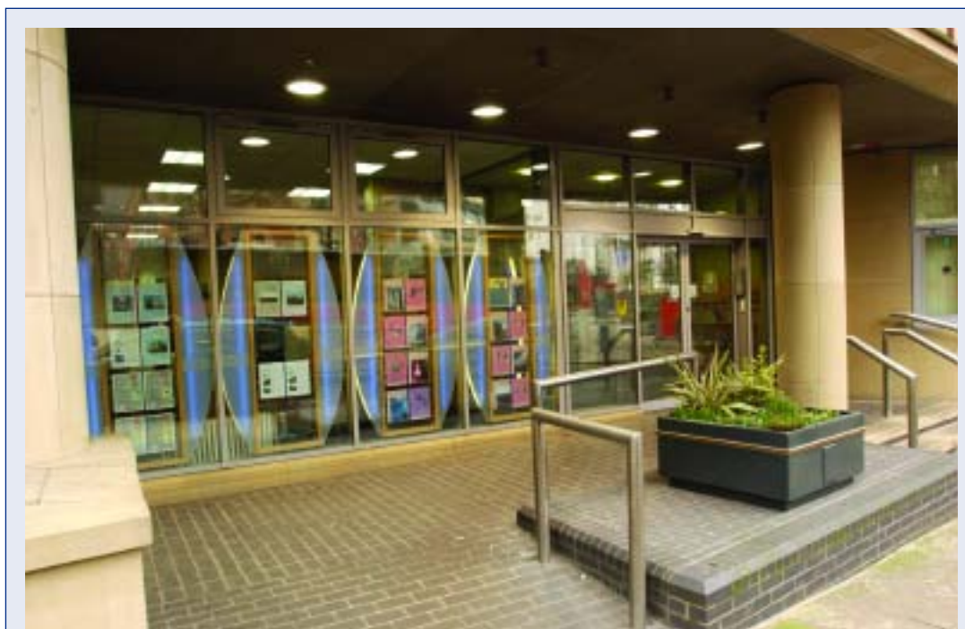
Flat or sloping or ramped access and automatic doors are necessary to allow access for disabled people.
