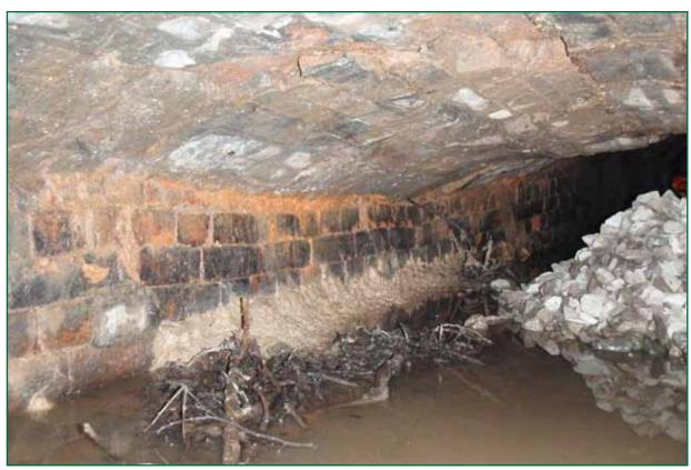
*Figure 9: Deformation to roof of deck E and leaning north abutment looking upstream (photograph courtesy of Amey)*
