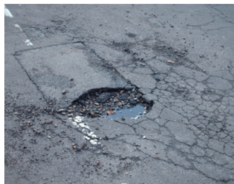
Pothole on previously repaired surface, image courtesy of Stephen Child Consultancy
