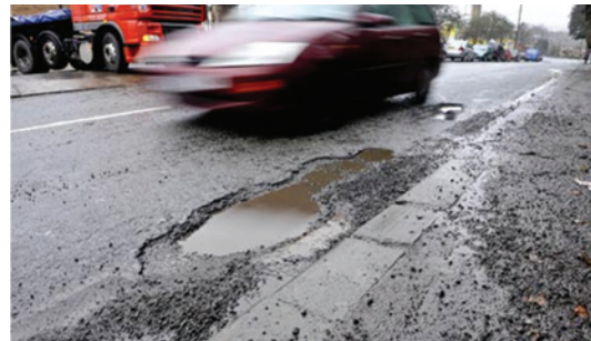
Water filled pothole near kerb, image courtesy of NHT Network
