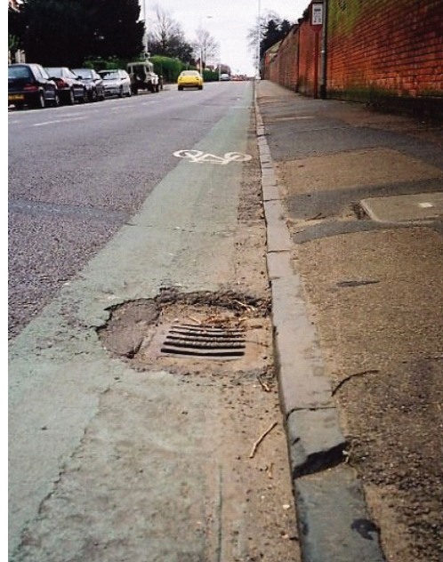
Damage surrounding drain cover, image courtesy of Well-maintained Highways
