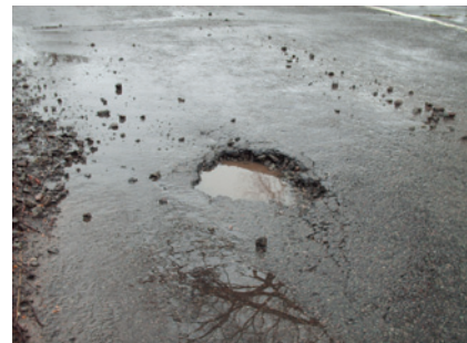
Severe pothole in carriageway, image courtesy of Stephen Child Consultancy
